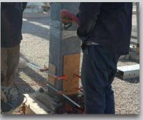
Fill the inside of the column with grout
